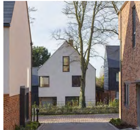
Framed view towards feature gable with staggered windows
