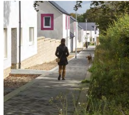
Permeable block paving
