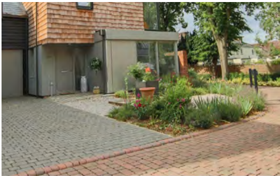
Permeable block paving in different colours to define spaces for parking.
