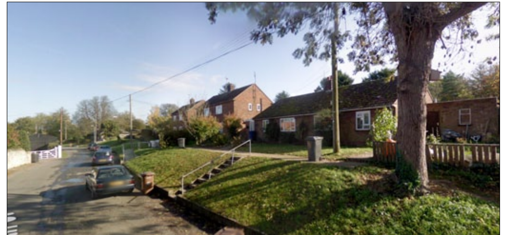
Local authority built housing on North Street
